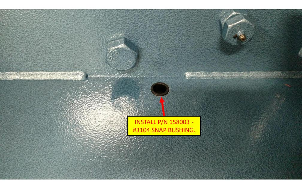
IF NOT ALREADY INSTALLED, REMOVE KNOCKOUT PLUG FROM ELECTRICAL BOX AND INSTALL P/N 158003 - #3104 SNAP BUSHING.
